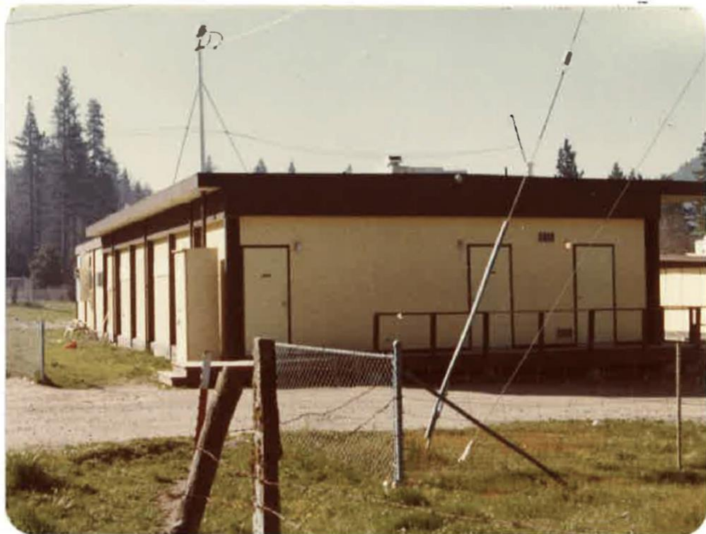
The north end of the Speed-Space building showing the entrances of the restrooms and the custodial storage room.
