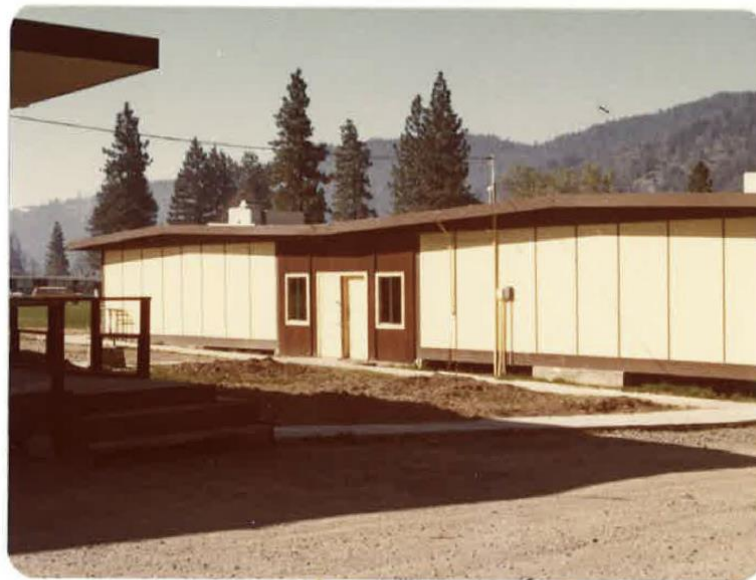
View of the student locker room which was constructed between the two Vinnell Corporation building.
