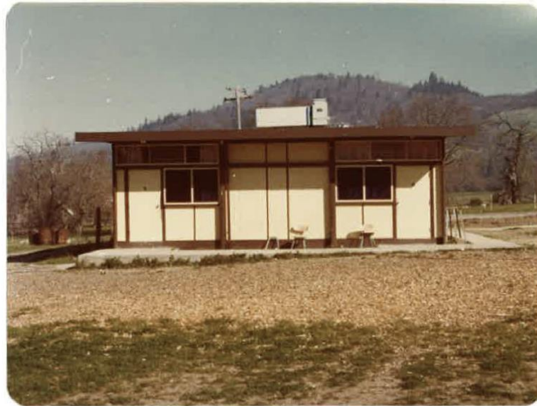
The Vinnell Corporation building containing the two classrooms for the social studies and math and science programs.
